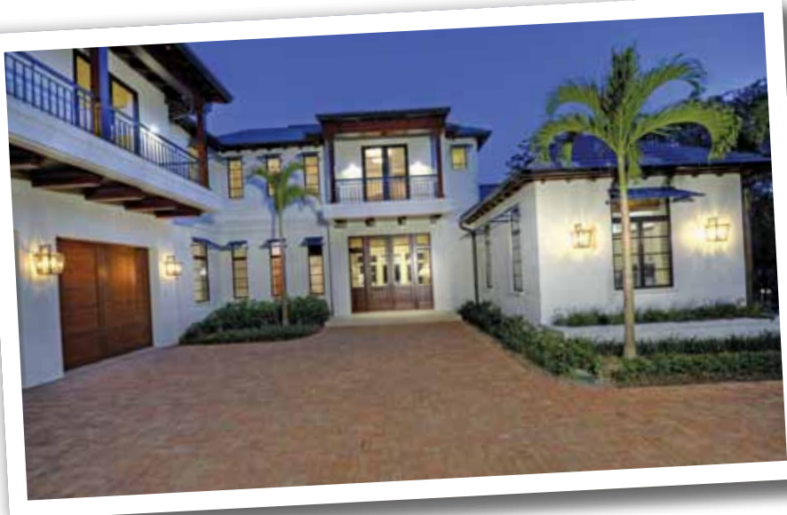
The influence of West Indies architecture is apparent in this design by Kukuk Architecture & Design. Built by A. Vernon Allen Builder, the front exterior features kerf corner columns, decorative rafter tails and beams together with Bahamian blue shutters.
